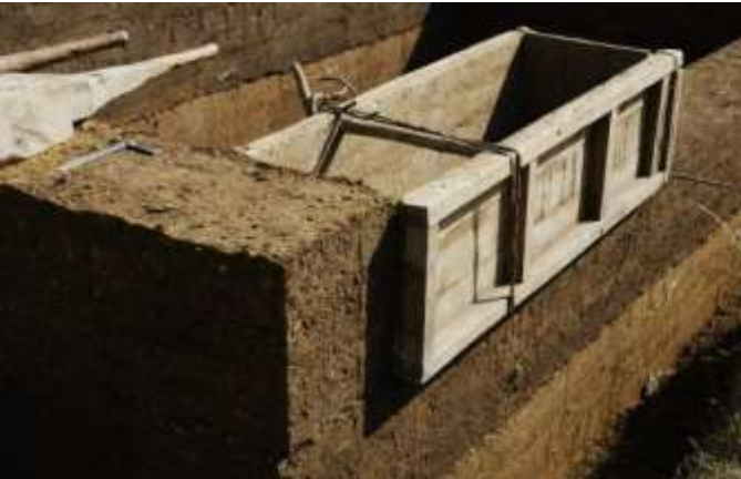
Rammed earth technique developed by Mrinmayee Bangalore Earth is rammed in a smaller blocks of 2 feet length, using formwork which can easily be installed and shifted to adjacent sections of the wall
