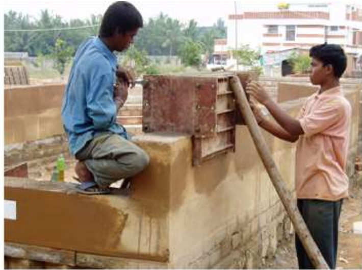
Rammed earth technique developed by Mrinmayee Bangalore Earth is rammed in a smaller blocks of 2 feet length, using formwork which can easily be installed and shifted to adjacent sections of the wall
